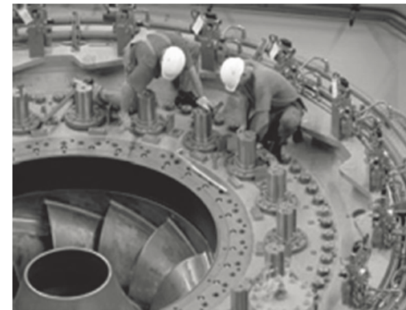
Figure 12.33 Runner and top cover for pump turbine, Waldeck, Germany. (Courtesy of Voith Hydro.)
